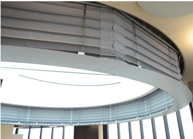
Figure 1: Images showing concertina Active Fire Curtain and a typical Active/Smoke Curtain
